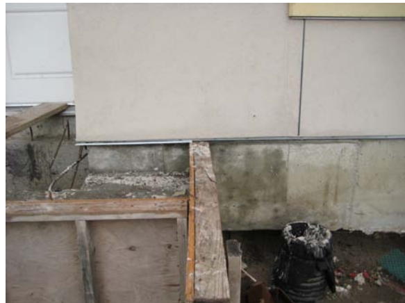
Vol. 4 – bldg 16 west elevation (SW corner), concrete foundation/slab and adjacent drain inlet.
