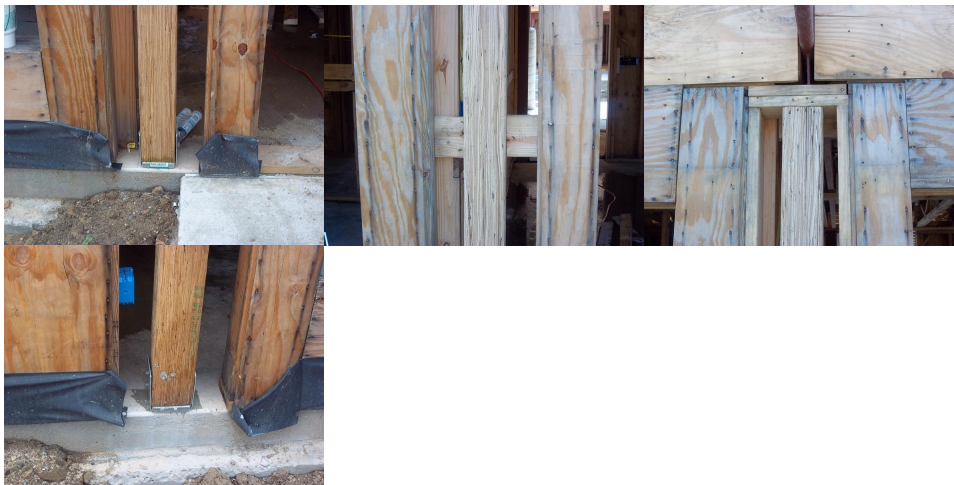
Items above show framing after post installation.
