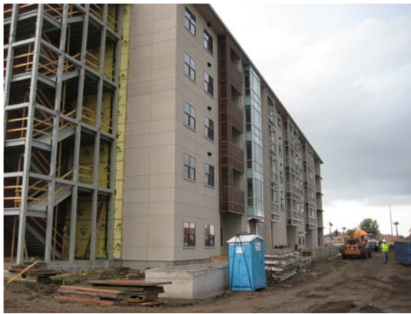
Vol. 4 – bldg 17 east elevation
