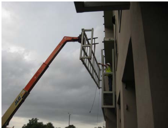
Vol. 4 – bldg 17 west elevation tube steel frame installation in progress
