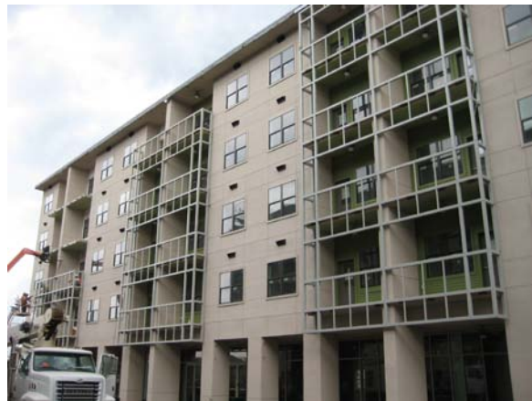
Vol. 4 – bldg 17 west elevation
