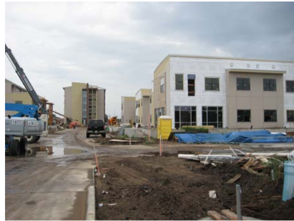
Vol. 3 – building B view from South
