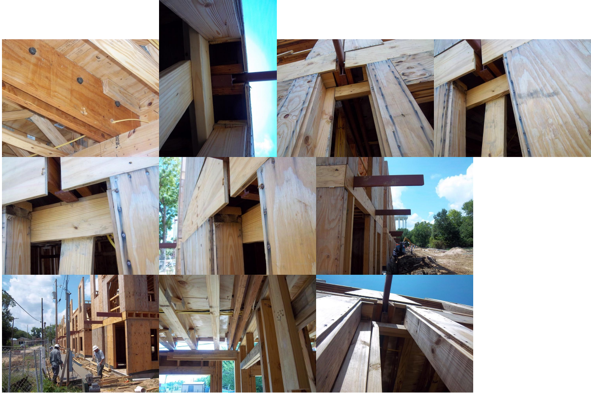
Items above show framing before post installation.
