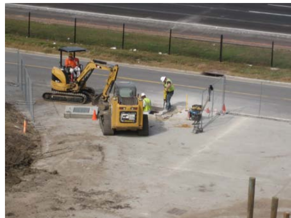
Volume 4 – rework of catchbasin at Northwest entry
