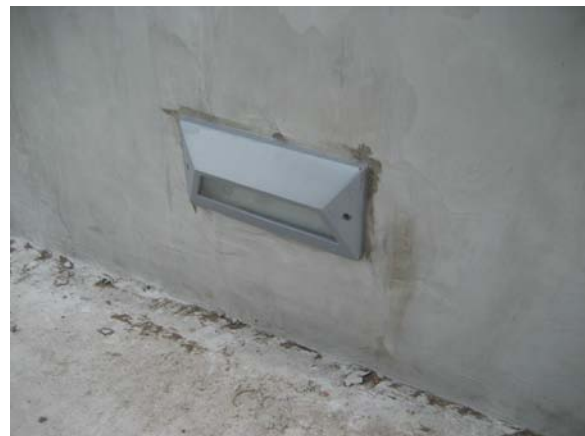
Vol. 3 – clear silicone smeared around fixture at concrete walls – unacceptable product and installation
