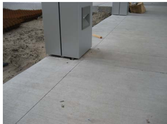
Vol. 4 – unacceptable gap at canopy metal panels.
