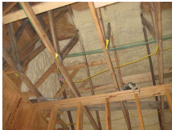
Volume 3 – spray foam installation in progress at roof deck
