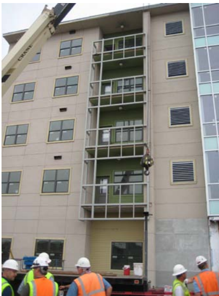
Vol. 4, Bldg 17 – installation of screen support framing remains in progress
