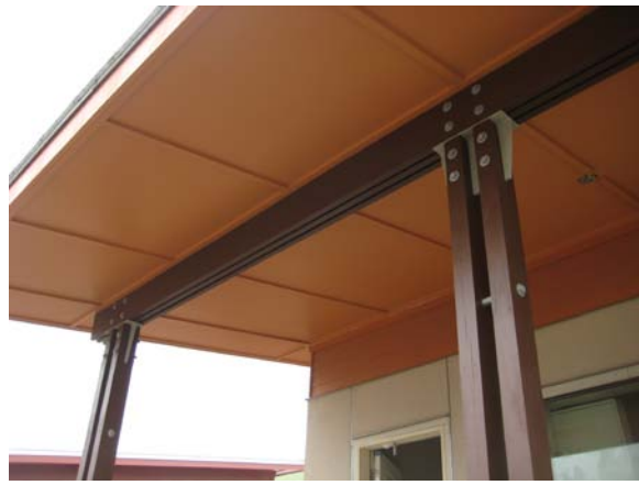
Opaque stain installation at vol. 2, bldg 1
