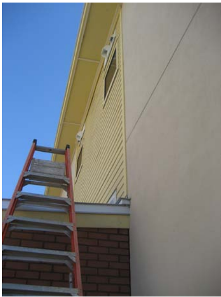
Volume 3 – joint between brick/siding/stucco
