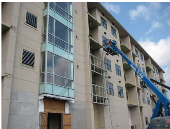
Volume 4 – building 17, screen support structure installation at balconies
