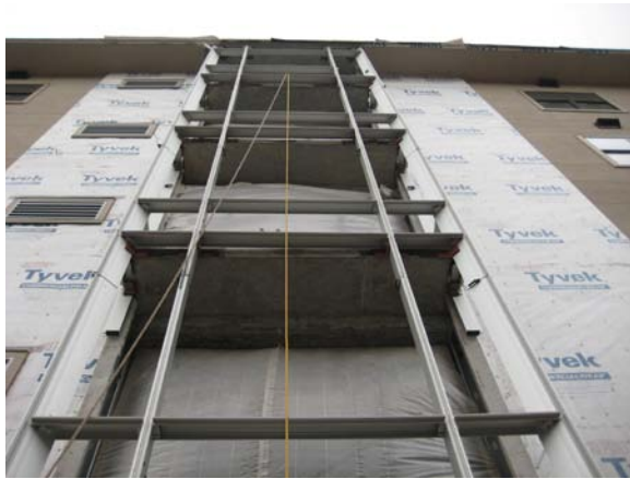
Bldg 16 curtainwall installation in progress
