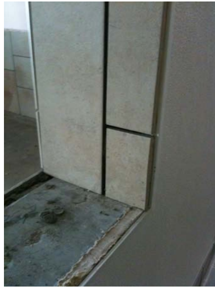
Volume 4 – kitchen 135 pass-through window. Tile alignment must be consistent along jamb.
