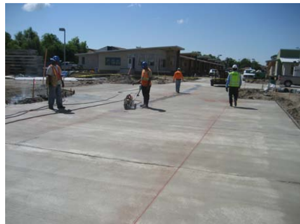
Village street, at volume 3 – sawcutting joints in progress
