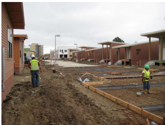
Forms and reinforcing for pavement between volume 1 and volume 2 (Village Street)
