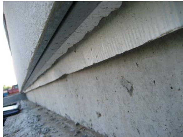
Volume 3 – bottom of wall condition at planters
