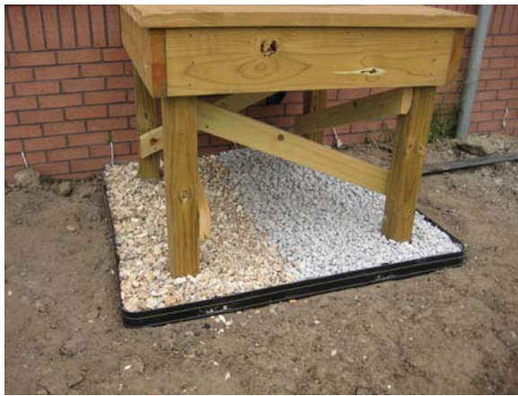
Gravel sample at vol. 1 HVAC platforms
