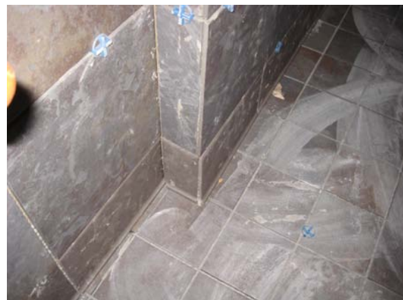
Vol. 4, bldg 17 - Ceramic tile installation at public toilets; factory formed outside corners required at cove base
