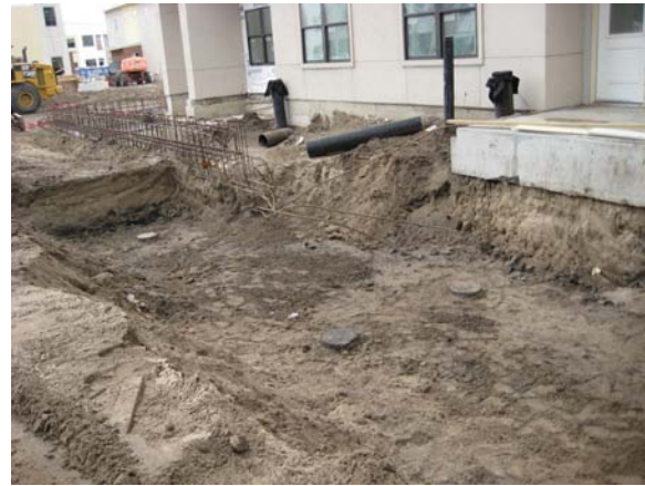
Excavation between bldgs 16 & 17 for site concrete
