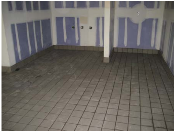
Quarry tile installation in progress
