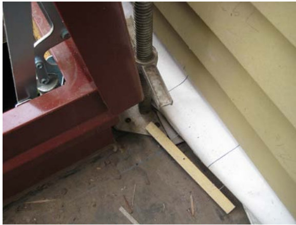
Volume 4 – space between roof hatch and wall is too tight for specified SBS Mod Bit flashing. Fluid applied flashing membrane will be applied
