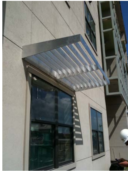
Vol. 4, bldg 17 – louvered awning mockup.
