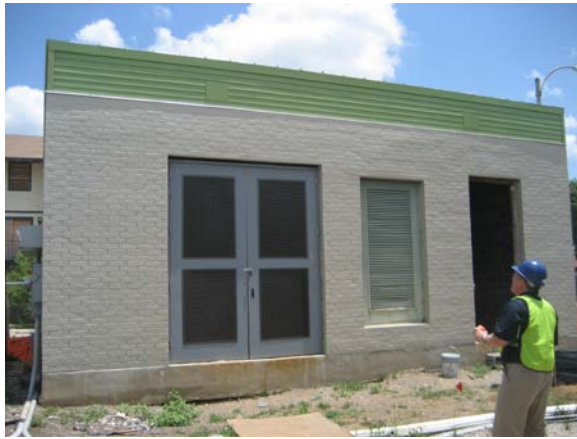
Electrical building, volume 1
