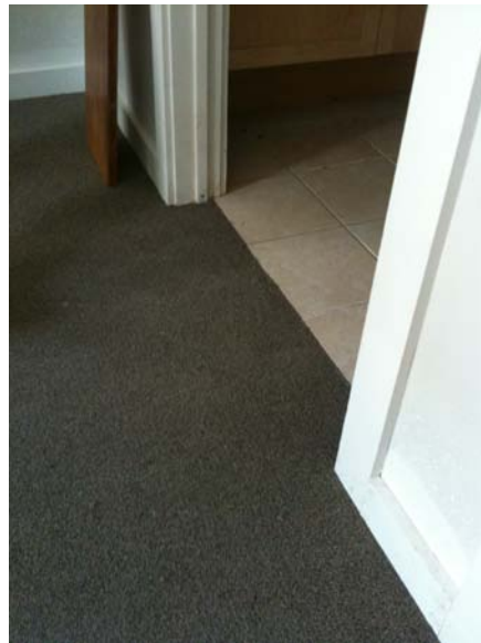
Volume 4 – carpet installation in bedroom
