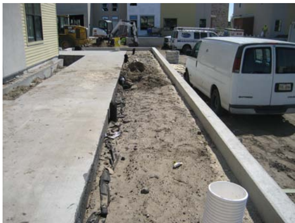
Volume 3 – drainage work in progress at planters
