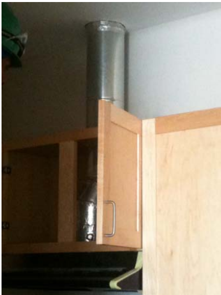
Volume 4 – mockup of exposed range duct
