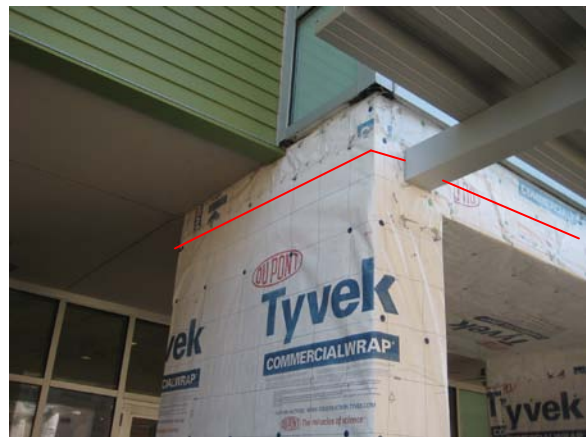
Vol. 4 - Joint required in metal panels as discussed to align with contractor proposed joint at column locations
