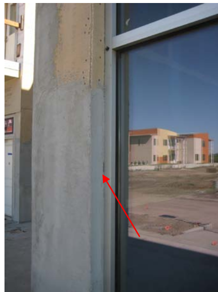
Vol. 3 – ¼" min. width sealant joint required between stucco and storefront.
