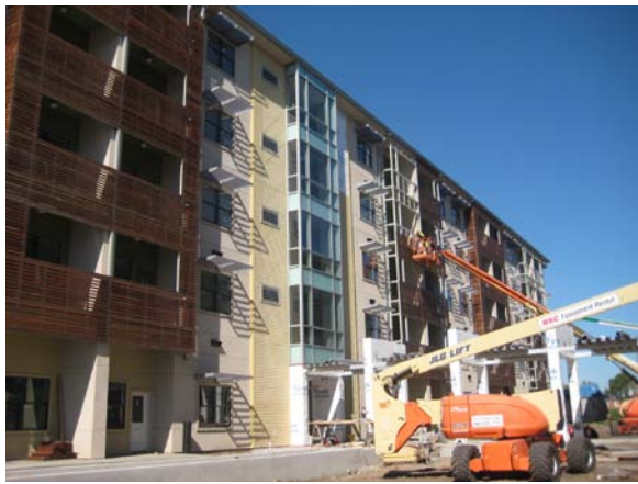
Vol. 4 – installation of wood slats in progress at balconies
