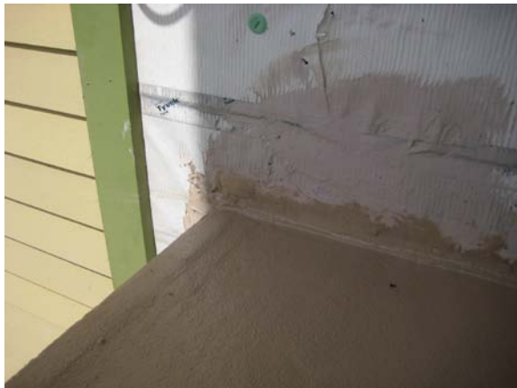
Volume 3 – deck coating sealed to Tyvek barrier at balconies.
