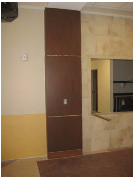
Vol. 4 – base different color from wall panels not acceptable
