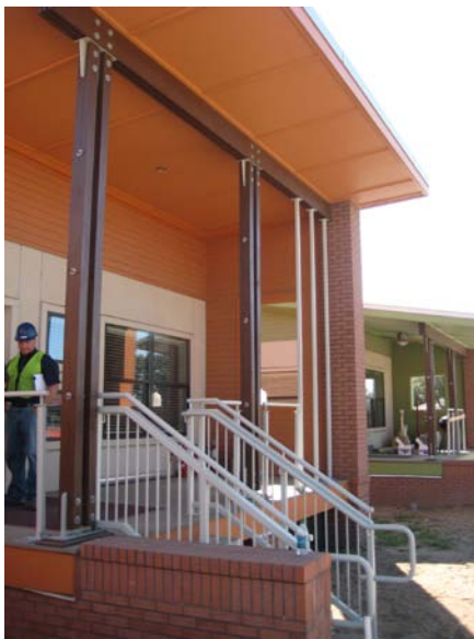
Vol. 1 – installation of wood slat support members and handrails
