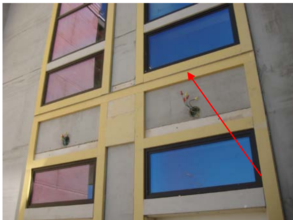
Volume 3 – flashing installed for canopy roof system
