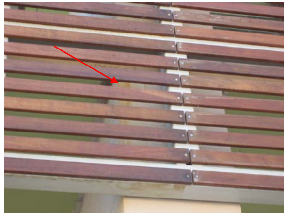
Vol. 4, building 16 – staining of steel and stucco still visible at col. D-10. Extensive washing has discolored Ipe wood. Remedial work required in this area.
