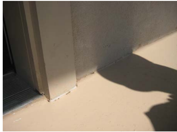
Volume 2 – deck coating sealed to stucco, no weeps
