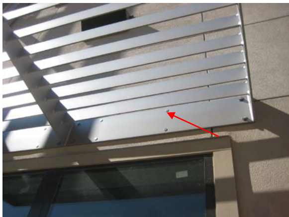
Plastic caps at vol. 4 awnings must be replaced with metal.
