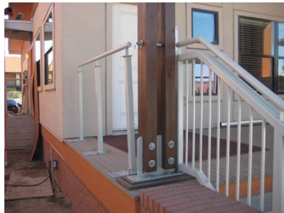
Vol. 1 – installation of guardrails without required top rail.
