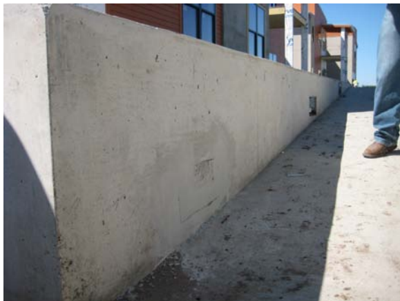
Remedial action at recessed lighting blockouts. Additional work required at wall.
