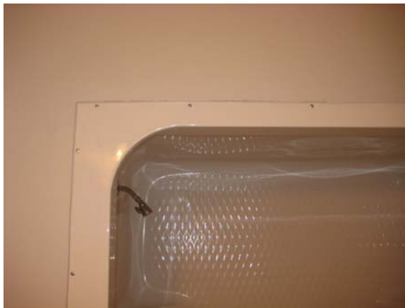
Exposed fasteners around perimeter of shower, volume 1, 2 typical
