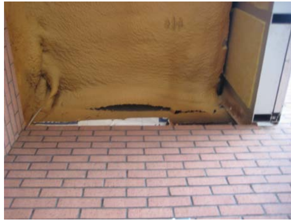
Repair of spray foam insulation required, North end of building 17, 1 st floor. Contractor shall identify method of flashing installation at base of curtain wall.
