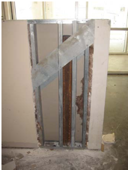
Tube steel support in knee wall, Building 17 salon
