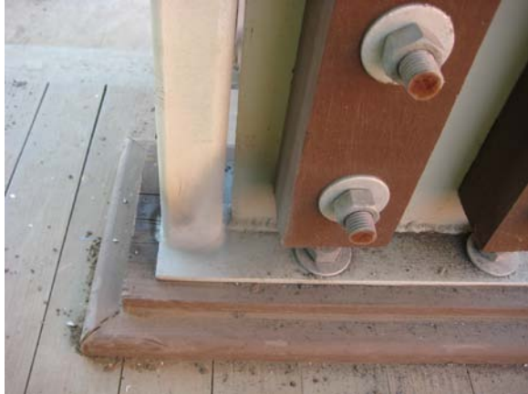
Vol. 1 – bldg 99 handrail connection mock-up
