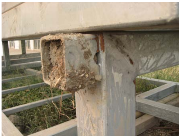
Connectors at volume 4 tube steel screen frames – rust, dirt present must be removed, steel galvanized and ptd.
