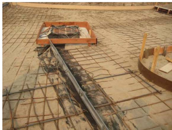
Contractor directed to center keyway on catch basin edge – south entry drive.
