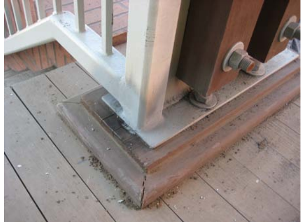
Vol. 1 – bldg 99 handrail connection mock-up
