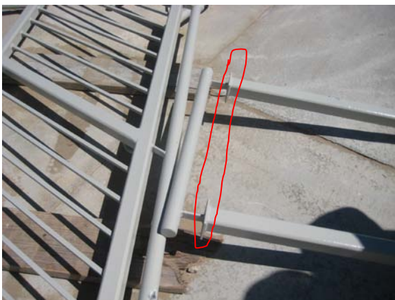
Flatbar at guardrails required to be continuous, typical for all guardrails to receive wood slats.
