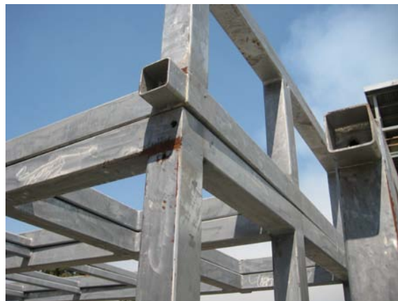
Rust present at connectors and joints of volume 4 tube steel screen frames – rust must be removed, steel galvanized and painted.
