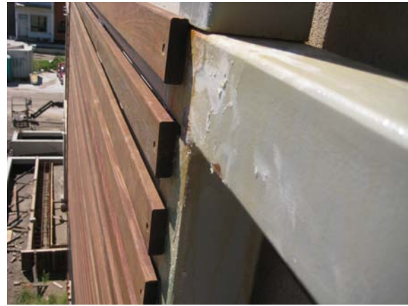
Staining on column D-10, Building 16 – residue on steel.
