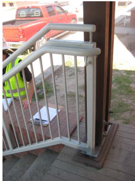
Vol. 1 – bldg 99 handrail connection mock-up
