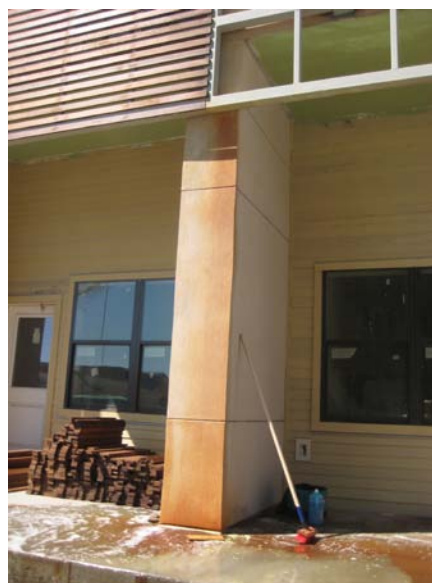
Staining on column D-10, Building 16
