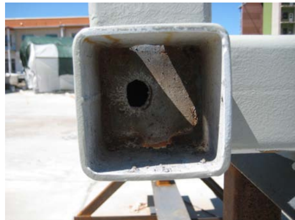
Tube steel sleeve connectors (volume 4) require additional rust removal, galvanizing, painting, typical.
