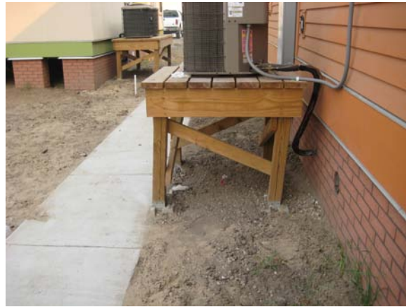
HVAC platform must be repaired/rebuilt due to lean
