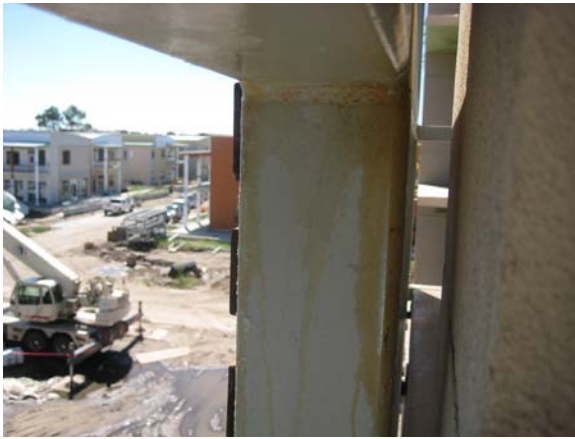
Staining on column D-10, Building 16 – residue on steel.
