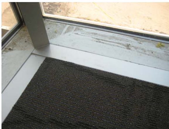
Volume 4 – curtainwall-to-slab closure; adjustment to break-metal required to address differing slab elevation along mullion, typical.
