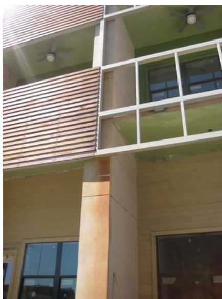
Staining on column D-10, Building 16
