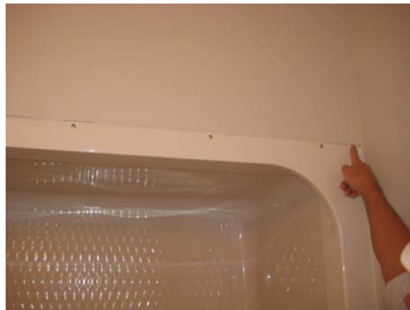
Exposed fasteners around perimeter of shower, volume 1, 2 typical
