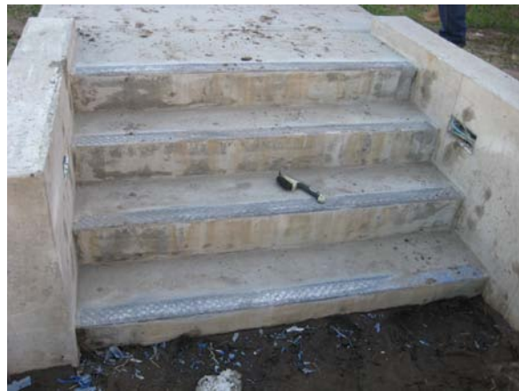
Rejected remedial action at volume 3 cast-in-place stair risers/treads.
