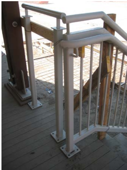
Vol. 1 – bldg 99 handrail connection mock-up; flat-bar at top of posts shall be continuous for each guardrail section.
