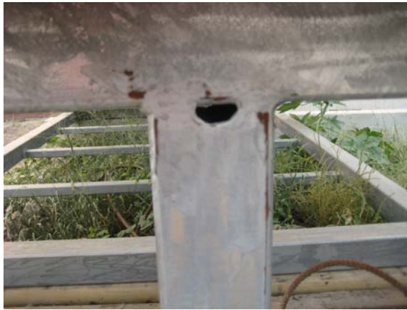
Rust present at connectors and joints of volume 4 tube steel screen frames – rust must be removed, steel galvanized and painted.
