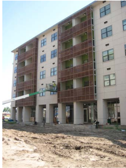
Vol. 4, bldg 17 – wood slat installation in progress.
