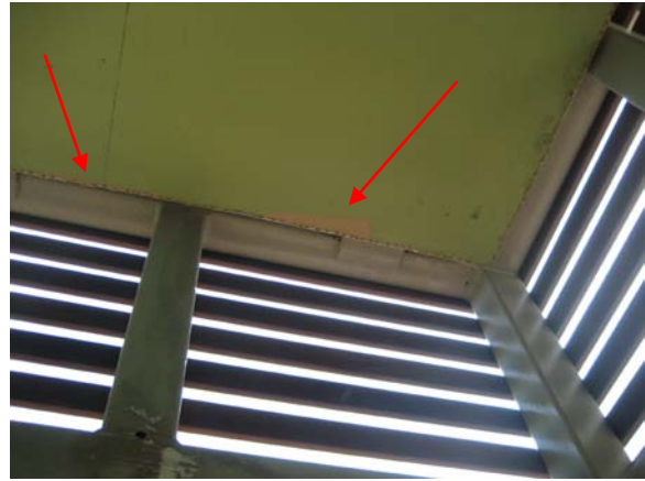
Vol. 4 – Bldg 17, drips and brush over at balcony ceiling from deck coating above.
