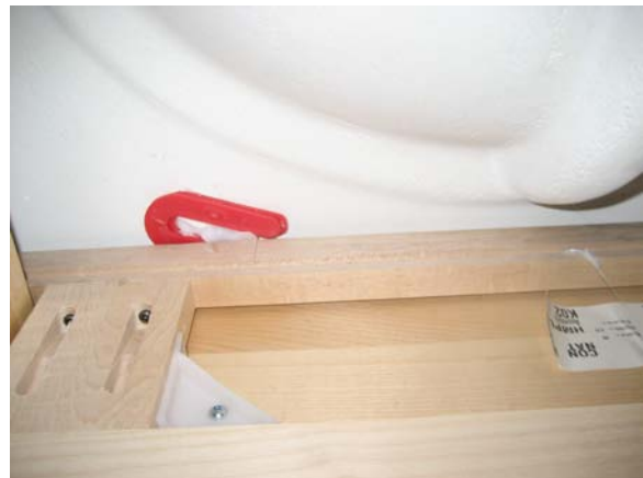
Vol. 4 – vanity top shims not acceptable (view from inside cabinet)
