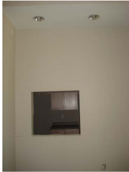
Volume 3 - Incorrectly placed recessed lights at kitchen pass-through
