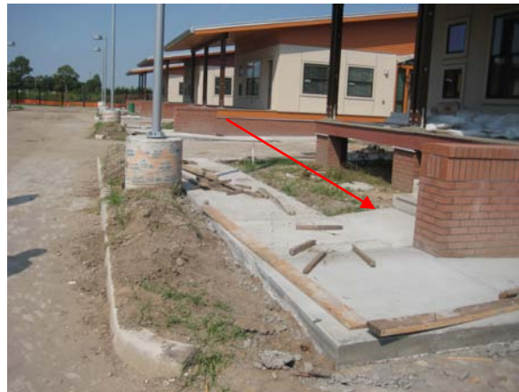
Improper slope at lower landing of entry steps
