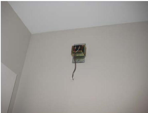
Exposed doorbell transformer, typical.
