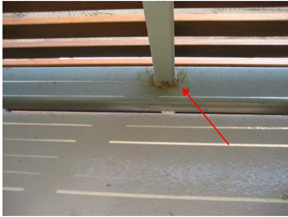
Vol. 4 – bldg 17 rust at base of intermediate screen support of balcony screen.
