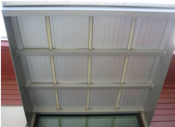
Prefinished steel or stainless steel roof clips required. Remainder of installation acceptable.
