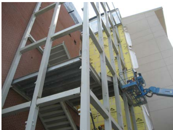
Vol. 4 – erection of steel stairs in progress, Bldg 17 north end.
