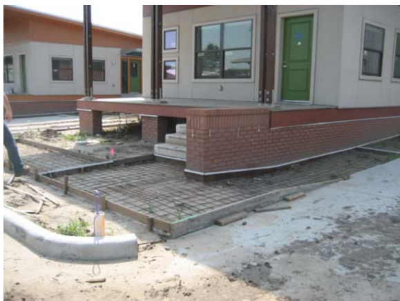
Vol. 2 – forms for sidewalk paving at Pecan Lane
