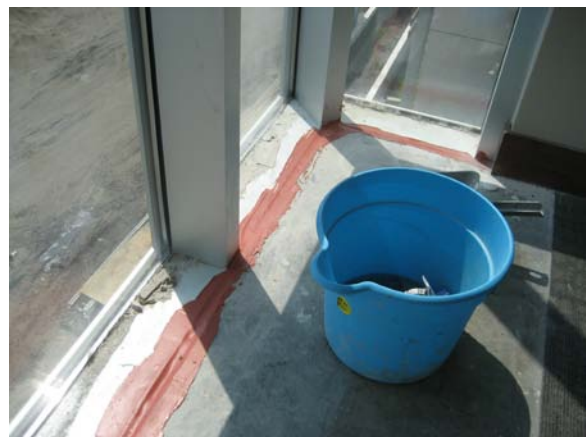
Vol. 4 – bldg 17 elevator lobby fire safing
