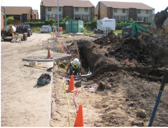
Conduit installation at Lake Forest entry
