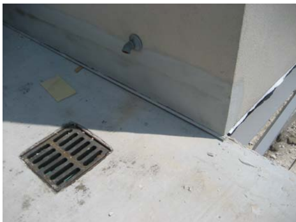
Vol. 3 – flashing installation acceptable, but still requires backer rod and sealant. Weep between stucco and flashing must be cleaned.
