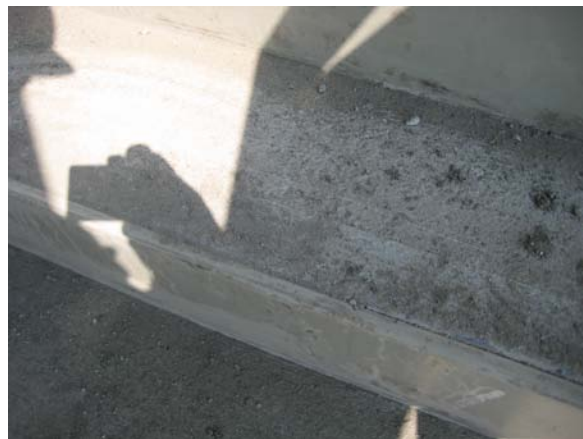
Volume 4 – stair tread concrete finish rejected
