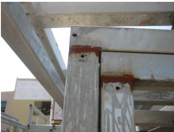
Repair needed at rusted connections for tube steel screen supports. Screens arrived unpainted.
