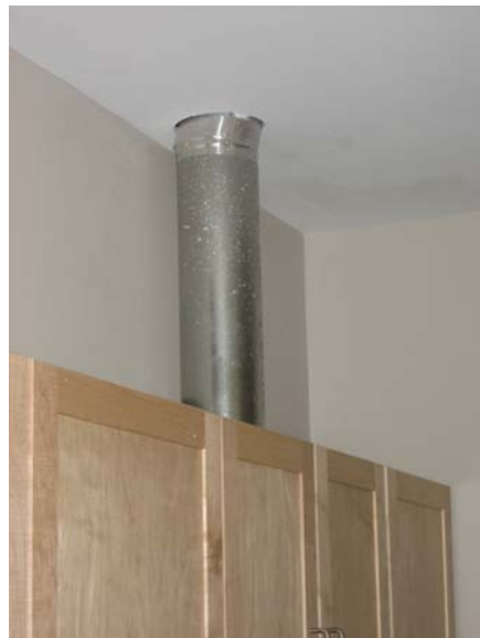
Vol. 4 – offset in range hood vent duct not acceptable to be left exposed, liner required to be installed.
