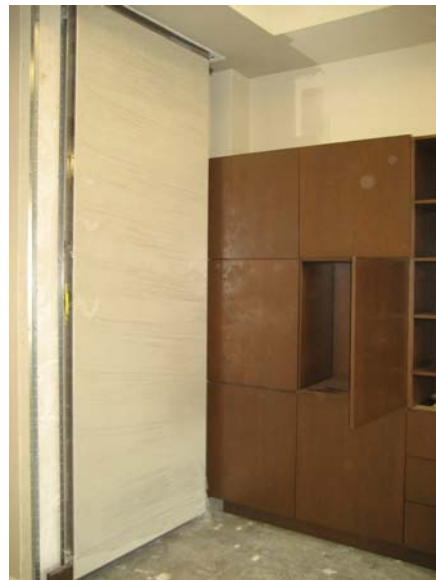
Vol. 4 – Library 130 millwork at North wall in conflict with operable partition.
