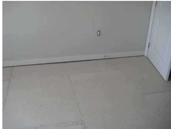
Unacceptable gap between floor and base, typical. (vol. 3 2 nd floor shown)
