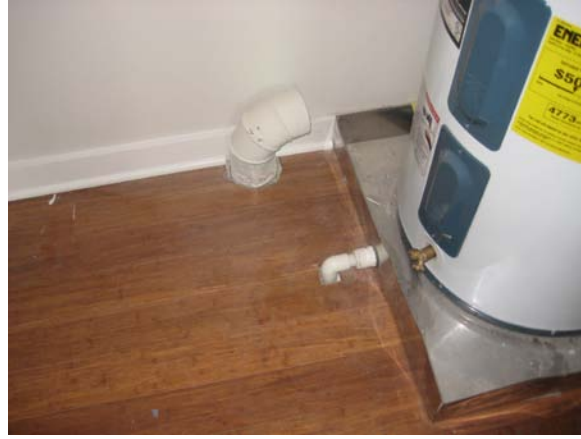
Trim required at exposed penetration of pvc through floor, typical (Vol. 2 shown)
