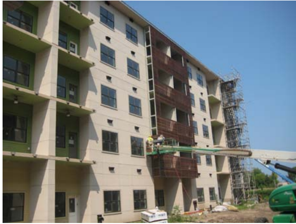
Volume 4 – Ipe installation at building 16, east elevation
