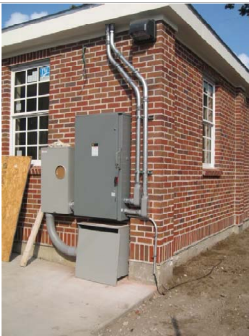
Electrical panel and meter on the rear corner of the building.
