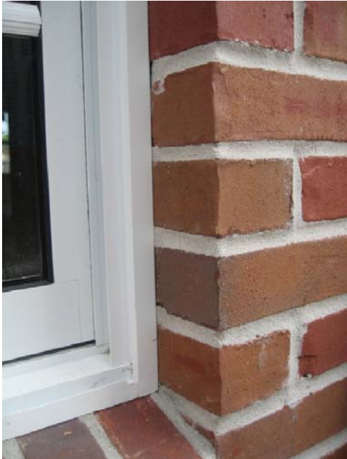
Sealant still needed around the exterior windows.
