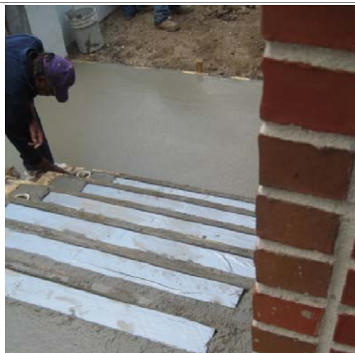
Concrete workers are finishing the stair treads at this time. Non-slip nosings are installed.
