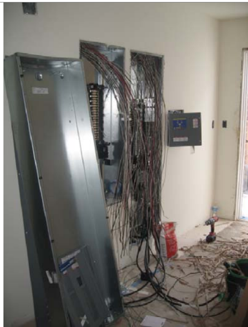
Work in progress on the interior electrical panel.
