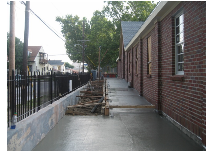
Concrete Ramp/Stair was poured this morning. Railing block-outs are in place.
