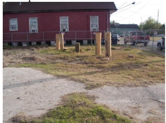
8 Test piles driven for reconstruction
