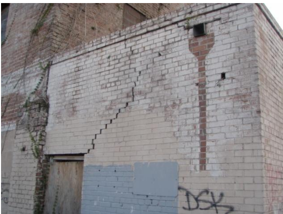
7 Stress cracks evident
