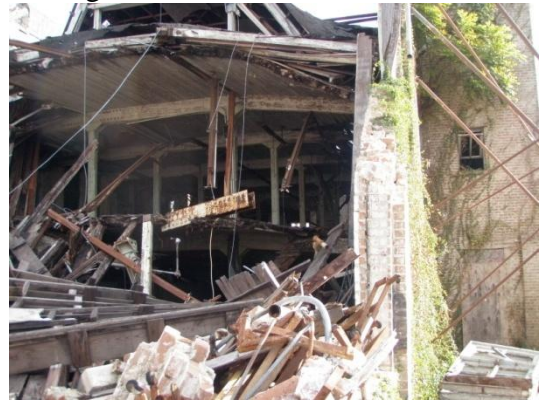
2 Building in state of collapse despite shoring efforts.
