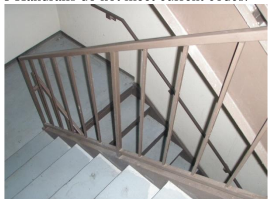
8 Handrails do not meet current codes.
