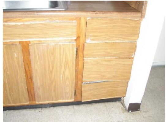
6 Cabinets need to be replaced.
