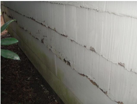
7 Siding has reached its maximum lifespan
