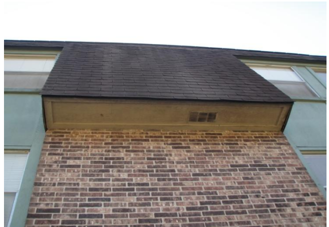
Soffit in need of repair/replacement.
