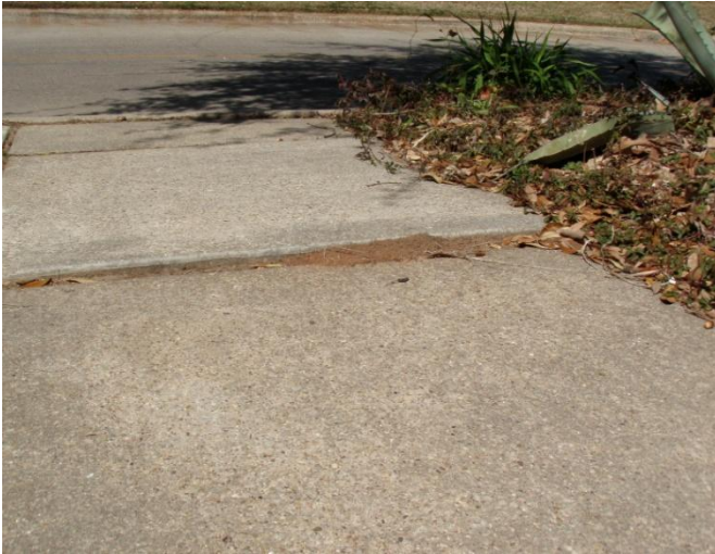
Slab settlement creating tripping hazards.
