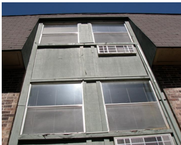
More decaying wood siding and trim at the window wall areas.
