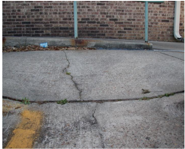
Concrete located at the drop off area in front is breaking down. Cracks in area of handicap parking.
