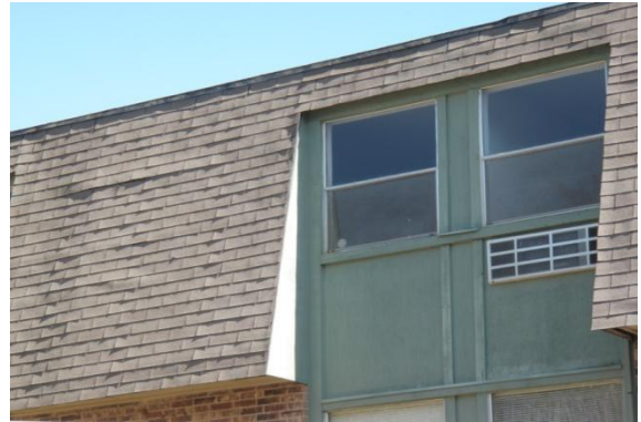
Emergency pull located in each bedroom & bathroom. Shingles in need of replacement
