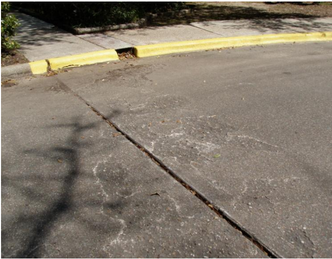
Concrete located at the drop off area in front is breaking down. Cracks in area of handicap parking.
