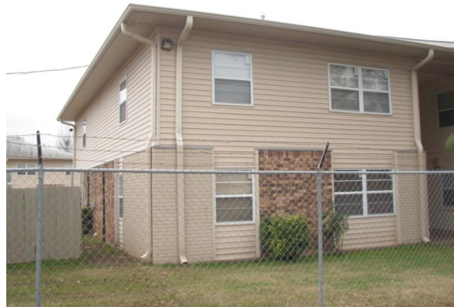
11. Water supply run thru siding allowing water intrusion. 12. Brick walls in fair condition - any brick throughout the site should be repaired & tuck pointed if needed. (typical throughout the site)
