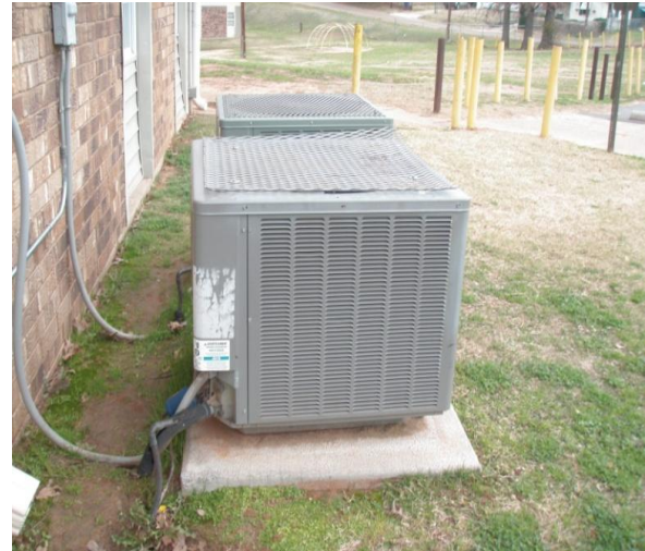
13. A/C slabs being undermined by water. Concrete slab at entrance failing. 14. Inefficient outdated HVAC A/C slabs not level, leads to inefficient operation & premature mechanical failure.
