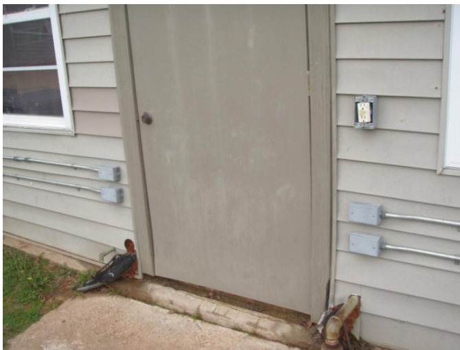
11. Water supply run thru siding allowing water intrusion. 12. Brick walls in fair condition - any brick throughout the site should be repaired & tuck pointed if needed. (typical throughout the site)
