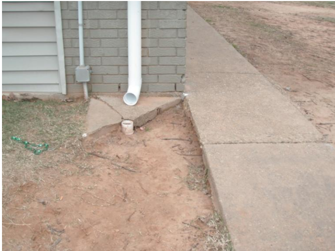
17. Gutter drain eroding away topsoil at walkway
