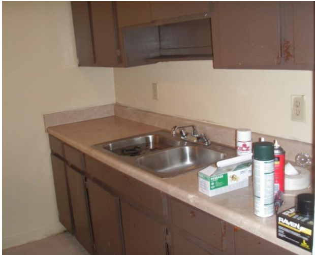
25. Kitchen area – Fixtures & plumbing need to be replaced along with failing cabinets & shelving. 26. Cooktop/stove and end of useful life and not energy efficient rated.
