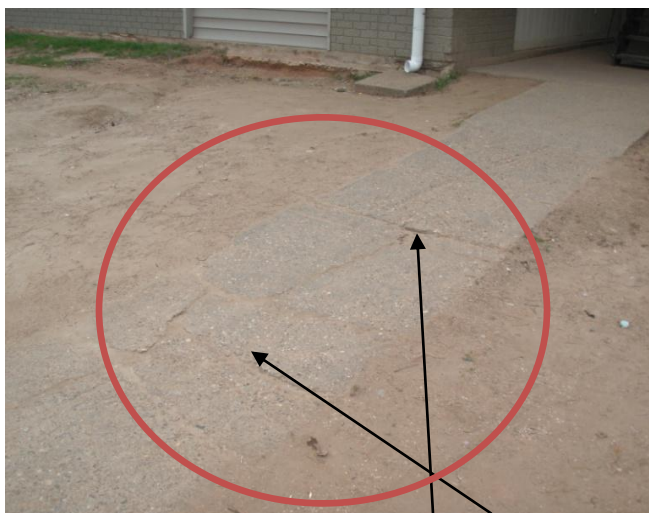
19. Accessible walkway failing. Cracks & settlement.
