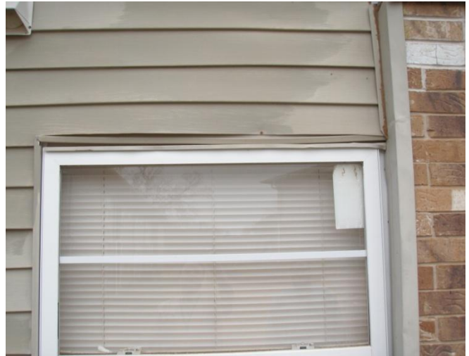
8. Siding above window warped allowing moisture intrusion
