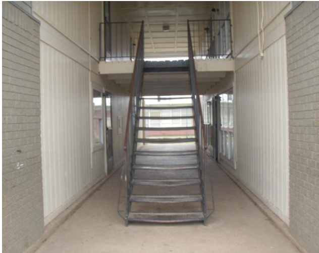
21. Bent stairs and handrails warrant repair or replacement.
