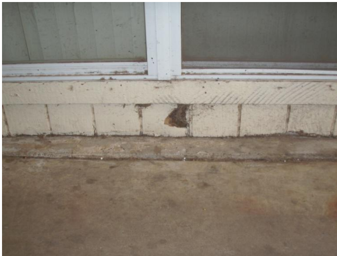
7. Siding under window failing
