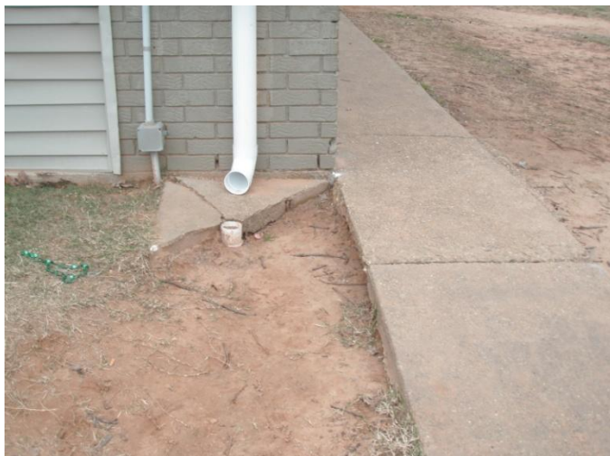
17. Gutter drain eroding away topsoil at walkway
