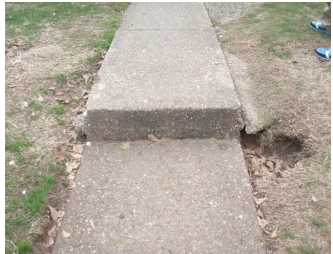
16. Sidewalk being undermined by water erosion
