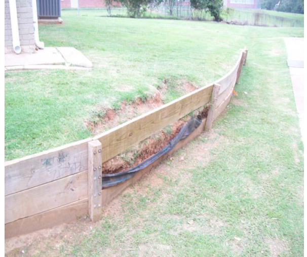
50. Failing retaining wall
