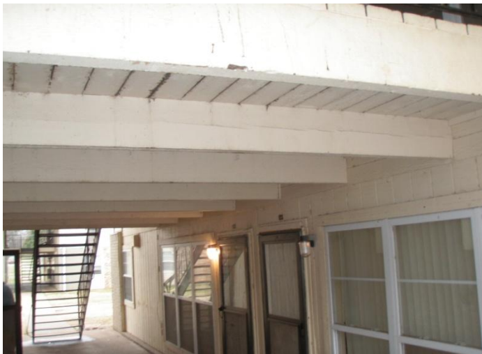
23. Wood structural beams in good condition at breezeways.
