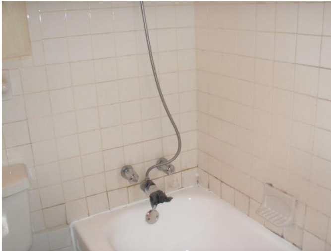
29. "Jerry Rigged" shower head. Shower fixtures throughout need replacing as well as most shower surrounds.
