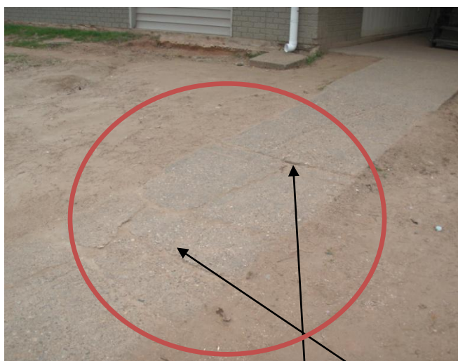
19. Accessible walkway failing. Cracks & settlement.
