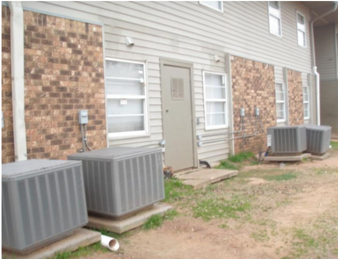
13. A/C slabs being undermined by water. Concrete slab at entrance failing. 14. Inefficient outdated HVAC A/C slabs not level, leads to inefficient operation & premature mechanical failure.
