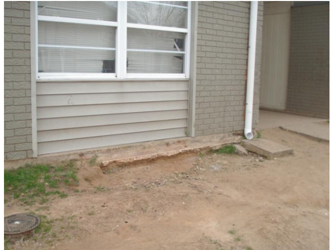
6. Soil erosion around slab area.
