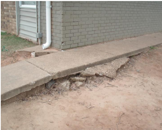
15. Accessible walkway failing.
