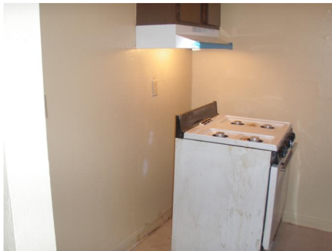
25. Kitchen area – Fixtures & plumbing need to be replaced along with failing cabinets & shelving. 26. Cooktop/stove and end of useful life and not energy efficient rated.
