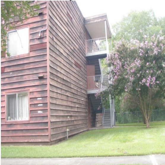
3 Siding has reached its maximum lifespan and needs to be replaced.
