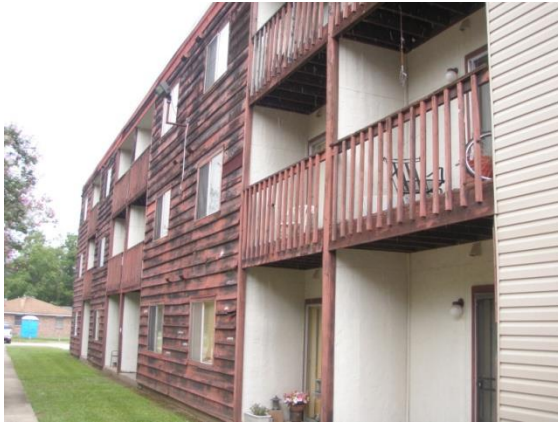
3 Siding has reached its maximum lifespan and needs to be replaced.
