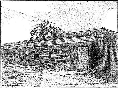
Exterior View of Subject
