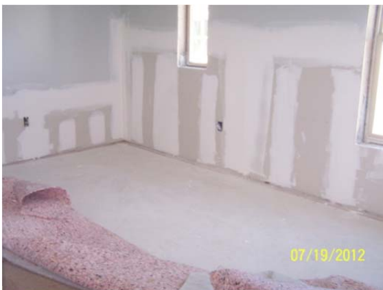
7 Drywall being finished Bldg #2
