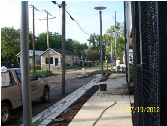
8. Landscaping being installed.
