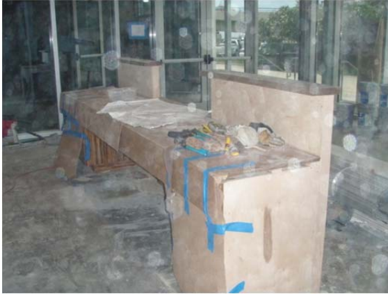
3 Receptionist desk being installed A.C.
