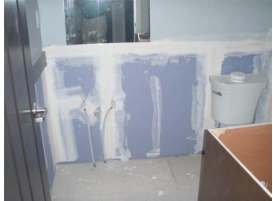
6 Drywall being finished Bldg #2
