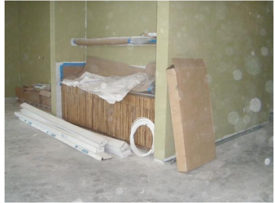
2 Interior nearing completion in the Activity Center.
