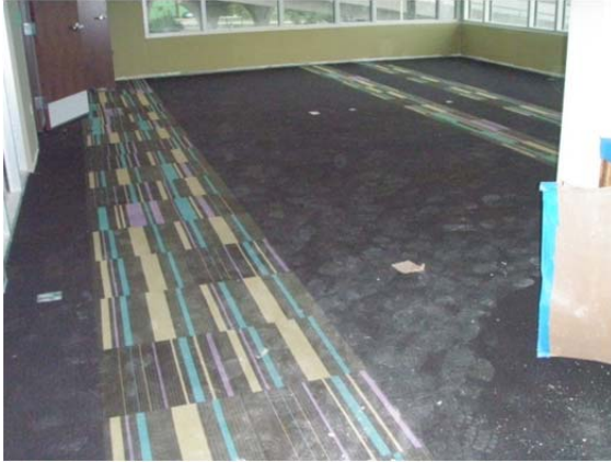
5 Flooring installed A.C.
