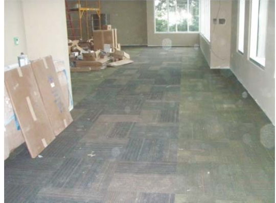
4 Flooring installed A.C.
