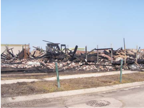
1 Debris on neighboring property
