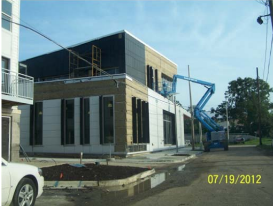
1 Exterior skin being installed A.C.
