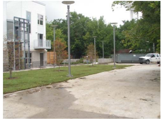
2 Landscaping being installed residential.
