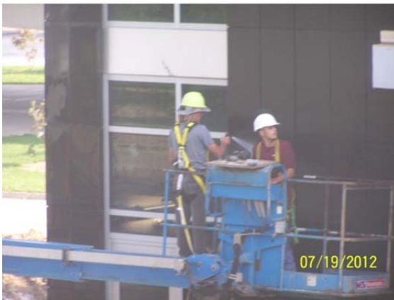
3 Installed skin being cleaned at A.C.
