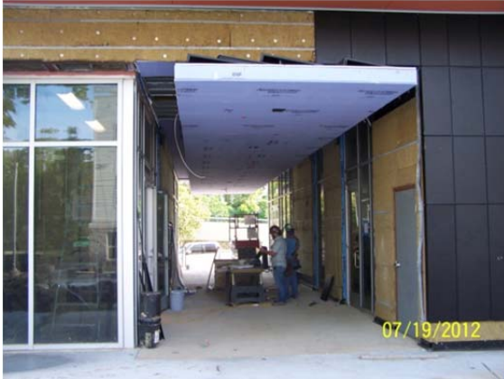
5 Panels being cut for installation at A.C.
