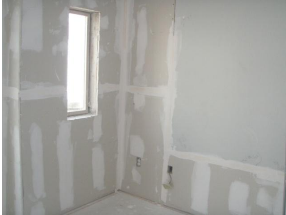
3 Drywall reinstall continues in Bldg #2.
