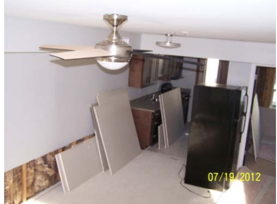
6 Drywall being finished Bldg #2
