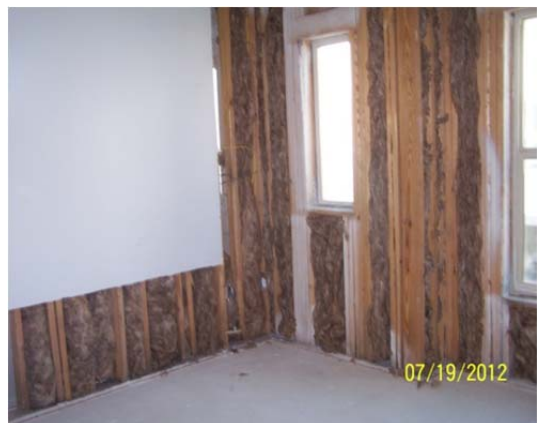
8 Walls awaiting Drywall at Bldg #2
