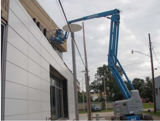
1 Exterior skin being installed A.C.
