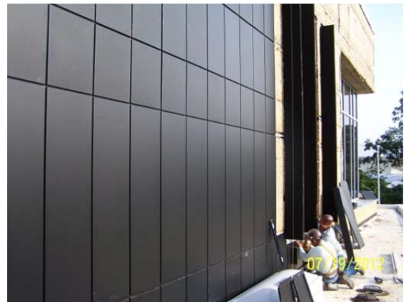
4 Craftsman installing panels at A.C.
