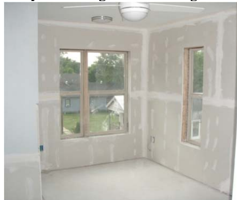
8 Drywall being finished Bldg #2
