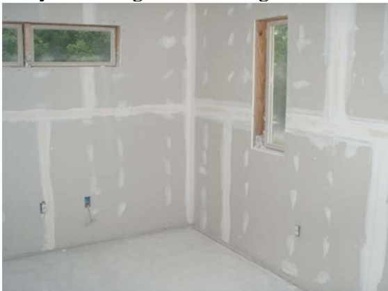
7 Drywall being finished Bldg #2
