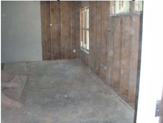
7 Final cleaning needed on Building #4.
