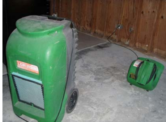
6 Final cleaning taking place in Building #3.
