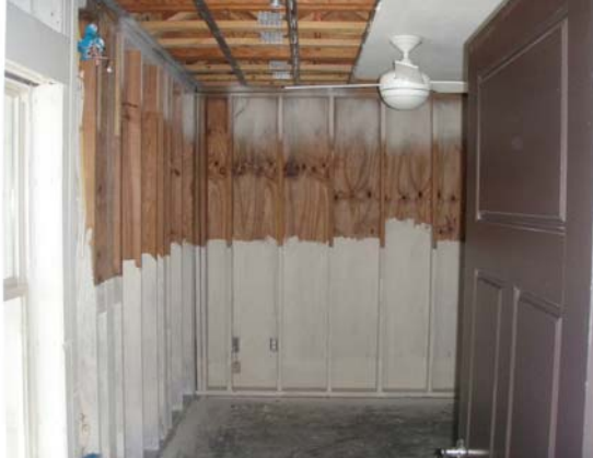
5 Clearance obtained on Building #2.
