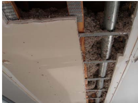
8 Extensive sprinkler corrections being made
