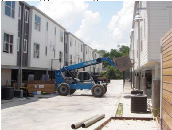
7 Demolition as part of the remediation plan taking place in bldg. 3.
