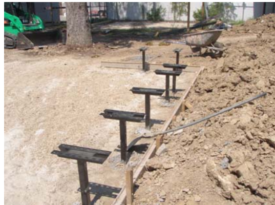
8 Benches being installed near Activity Center.
