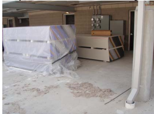
8 Drywall on site to refinish building #2.
