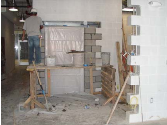
3 Elevator work being completed
