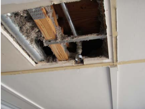
5 Sprinkler corrections being made
