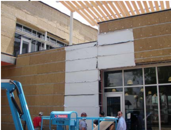
1 Exterior panels being installed on Activity Center
