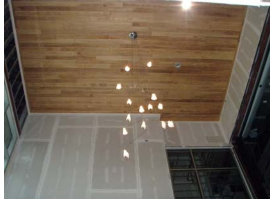
6 Forward progress continues
