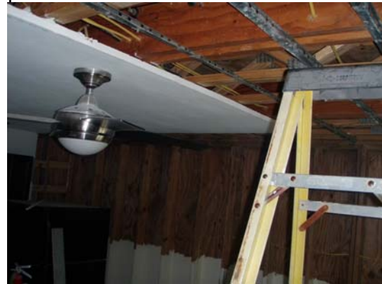
6 Extensive remediation work taking place
