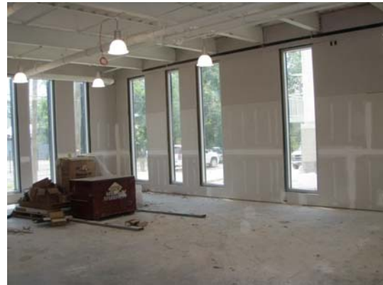
2 Drywall being finished in the Activity Center
