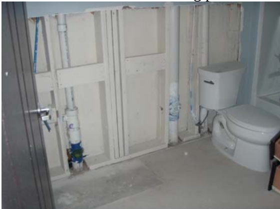
7 Extensive remediation taking place
