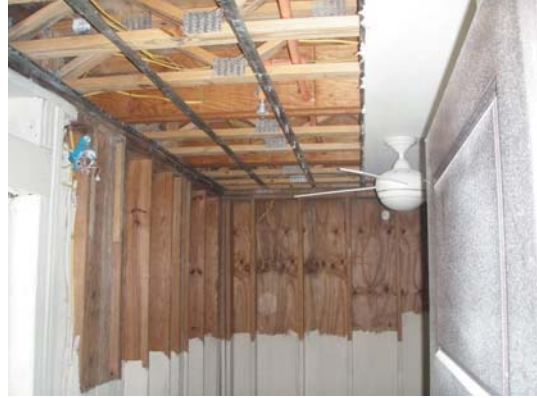
4 Extensive remediation taking place
