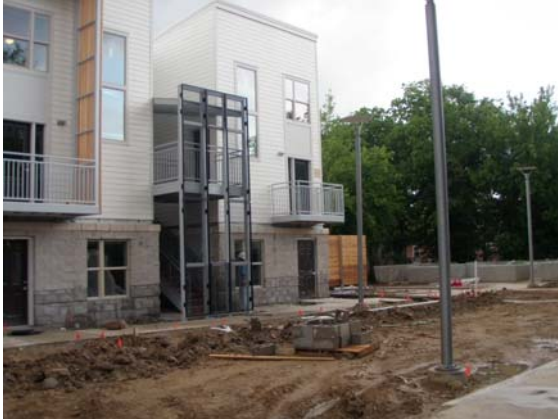
1 Masonry being brought to completion
