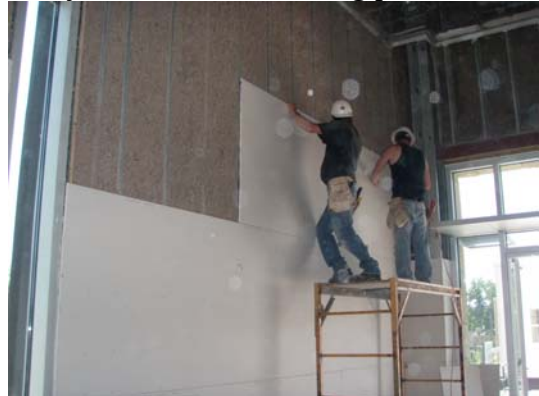
4 Drywall installation being performed
