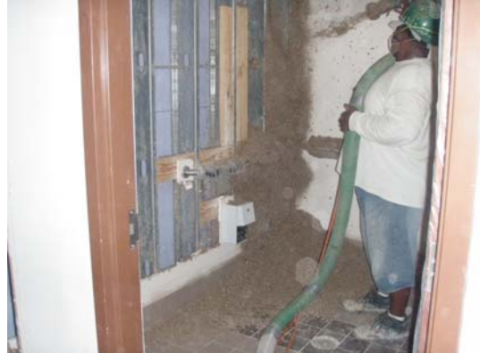
4 Insulation being reapplied in Activity Center
