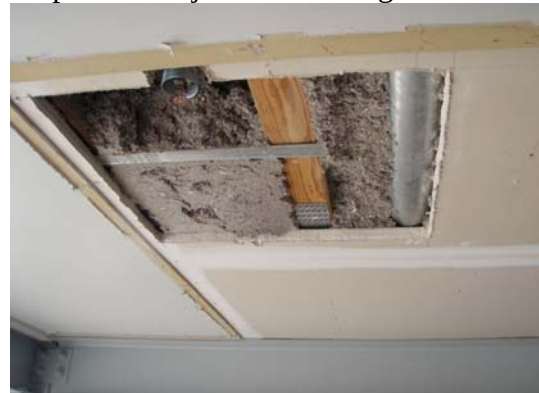
8 Sprinkler adjustments being made
