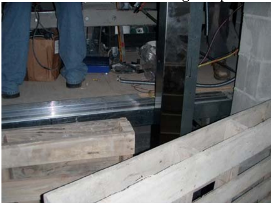
7 Elevator installation nearing completion
