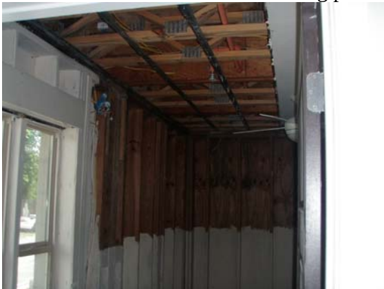
7 Extensive remediation work taking place
