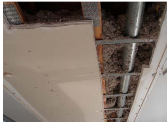
8 Extensive sprinkler corrections being made
