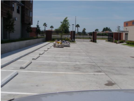
3 Construction Materials still on site
