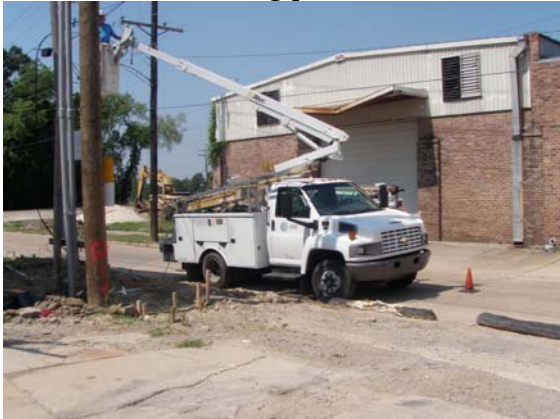
3 AT & T work being performed
