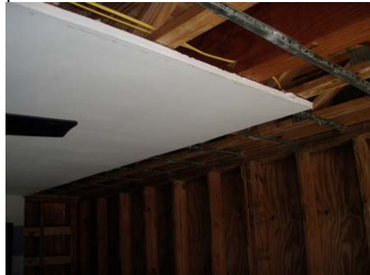
6 Extensive remediation work taking place
