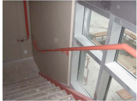
6 New grab bar installed with correct clearance.
