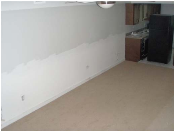
7 Drywall finished, ready to paint in residential units.
