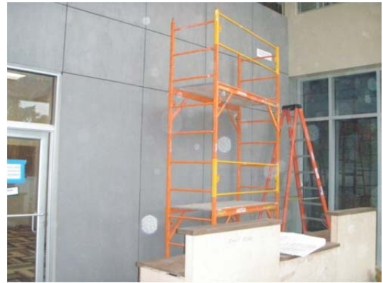
4 Finishes being installed in Activity Center.
