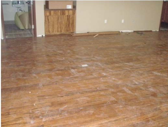
5 Wood flooring being installed in Activity Center.
