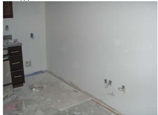
8 Drywall finished with floor reinstall taking place in residential units.
