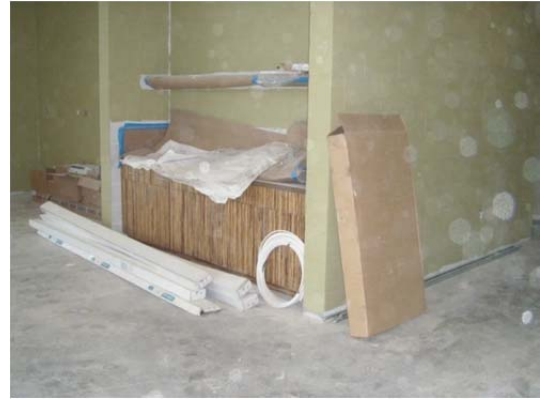
2 Interior nearing completion in the Activity Center.
