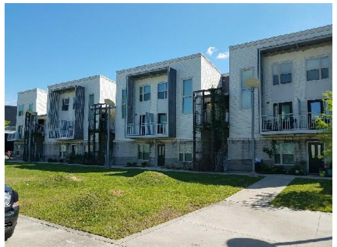
Typical exterior view of the subject
