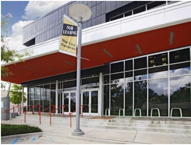
View of the subject Activity Center
