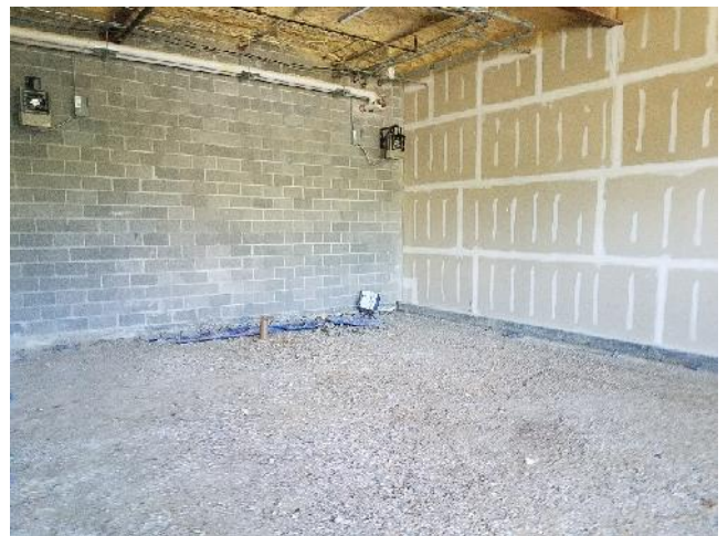
View of subject unfinished office space
