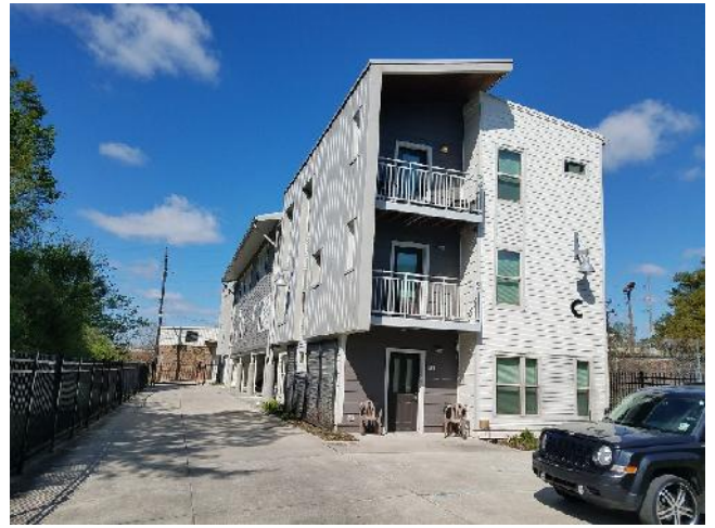
Typical exterior view of the subject residence buildings
