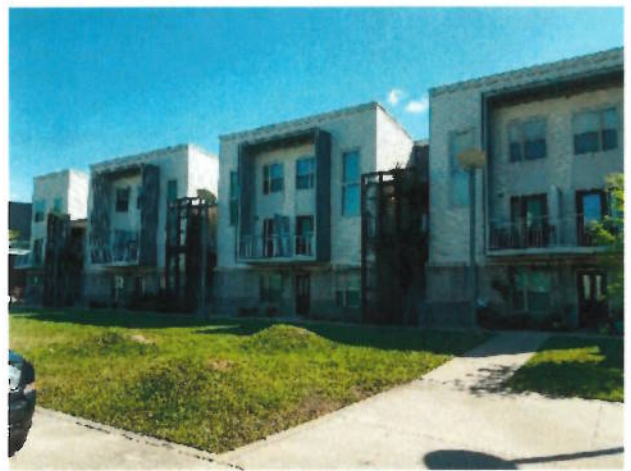
Typical exterior view of the subject
