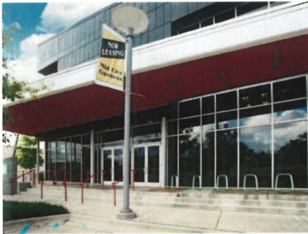
View of the subject Activity Center
