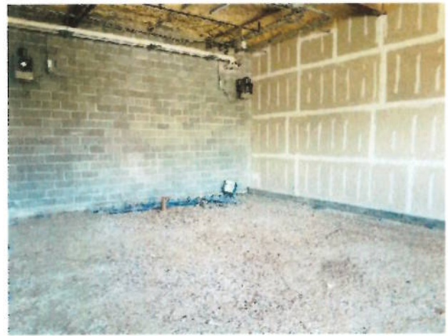
View of subject unfinished office space
